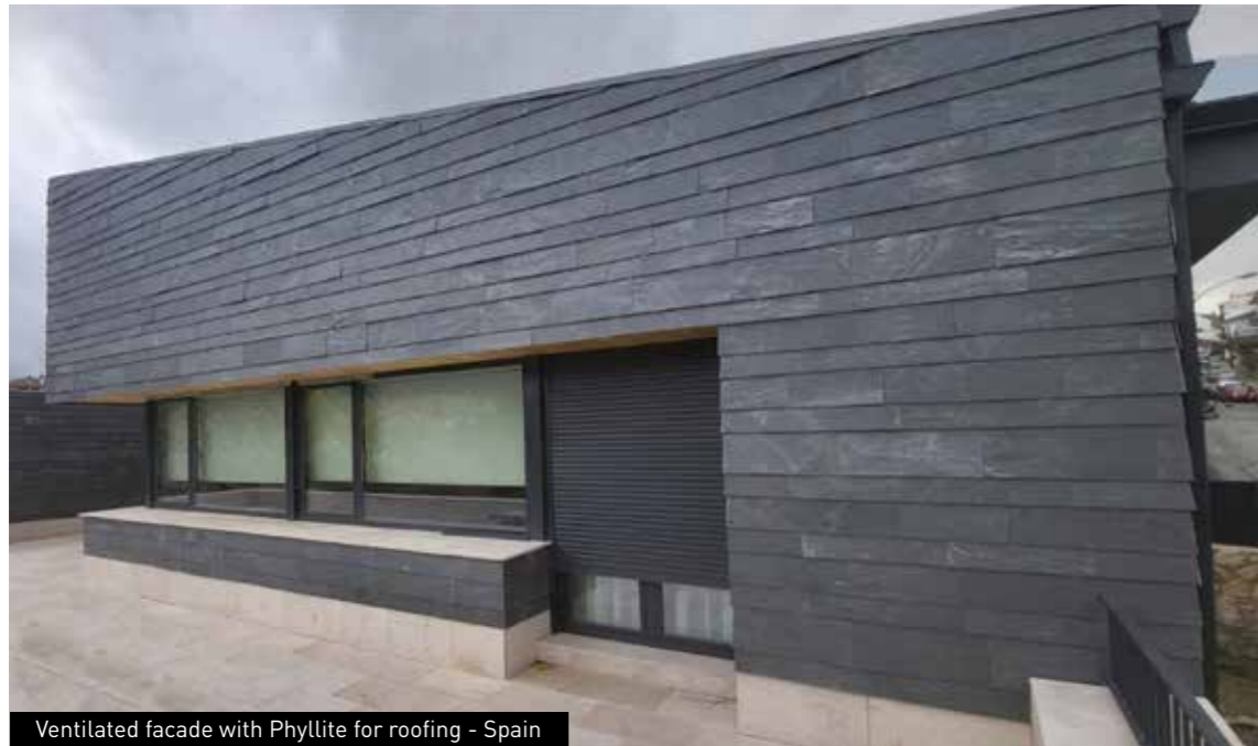
Ventilated facade with Phyllite for roofing - Spain
