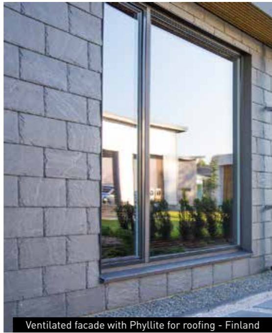
Ventilated facade with Phyllite for roofing - Finland
