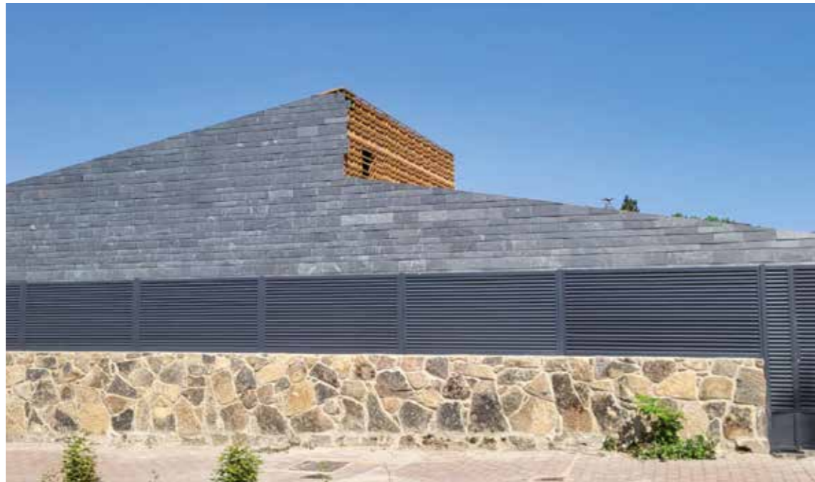
Ventilated facade with Phyllite for roofing - Spain
